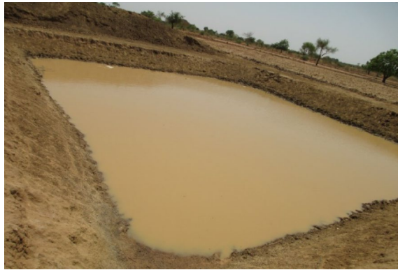
a) Pond with bottom and un-waterproofed walls on clay soil in Bam province
