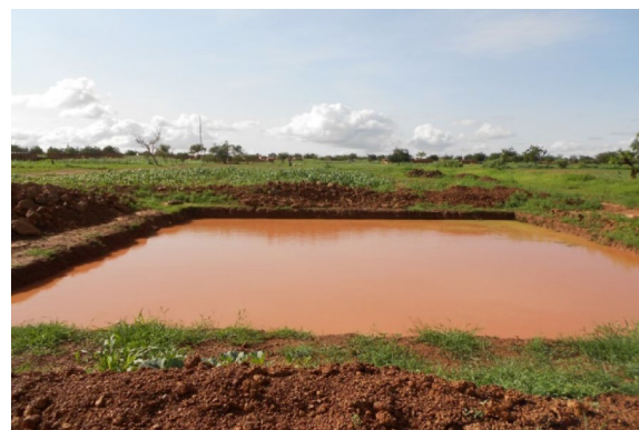
b) Pond with bottom and un-waterproofed walls on lateritic soil in Yatenga province
