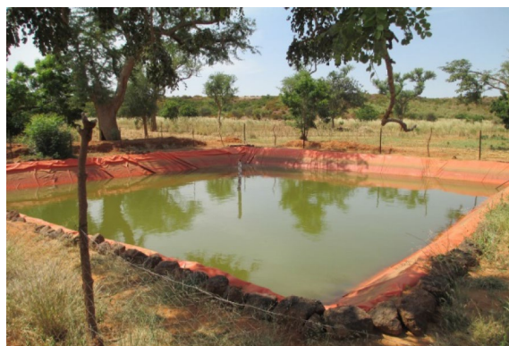
e) Pond with bottom and walls waterproofed with a tarpaulin in sandy soil in Bam province
