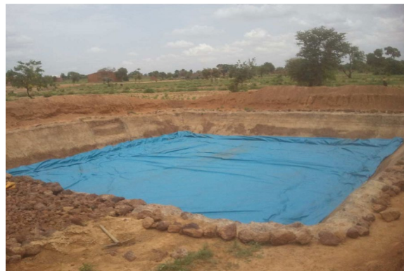
d) Pond with covered bottom and waterproofed cement walls in Yatenga province
